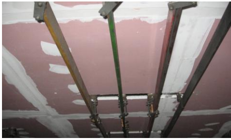
Figure 1. Substation in the basement of a school (10/0.4 kV, 1 × 1000 kVA)
